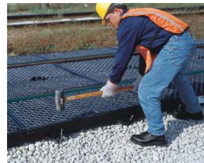
Side Pans are secured in place with 24" rebar fasteners. Typical installs require two pieces of rebar per Side Pan.
