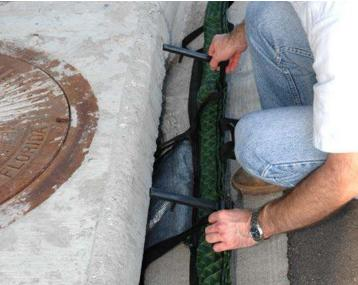
STEP 5: Install stabilizer arms (correct side is noted on grids STEP 6: Seal hook & loop fastener strips.
