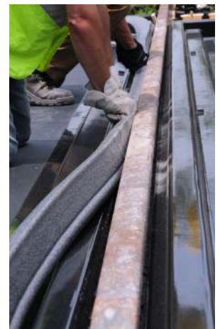
Optional rail side gaskets prevent leaking between rails and Track Pans.
